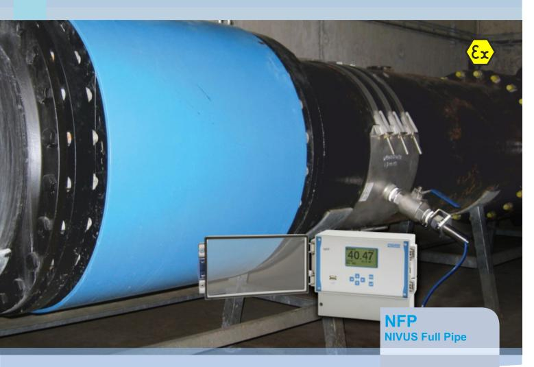
Flow Measurement for full Pipes
